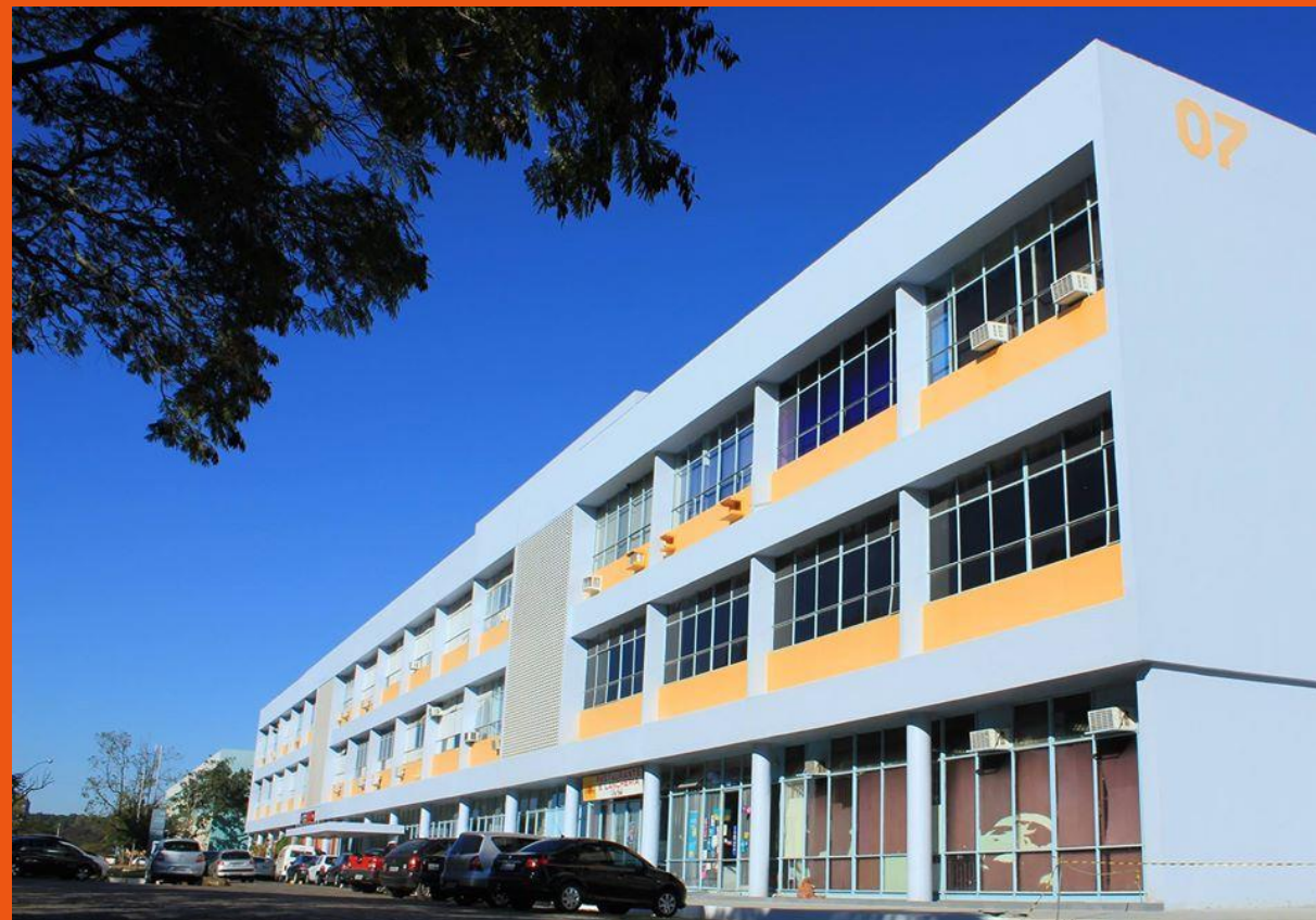
Fachada principal do CT/UFES
